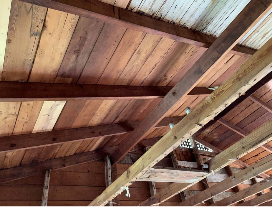
Pic 18– Randomly Placed Vertical Supports
