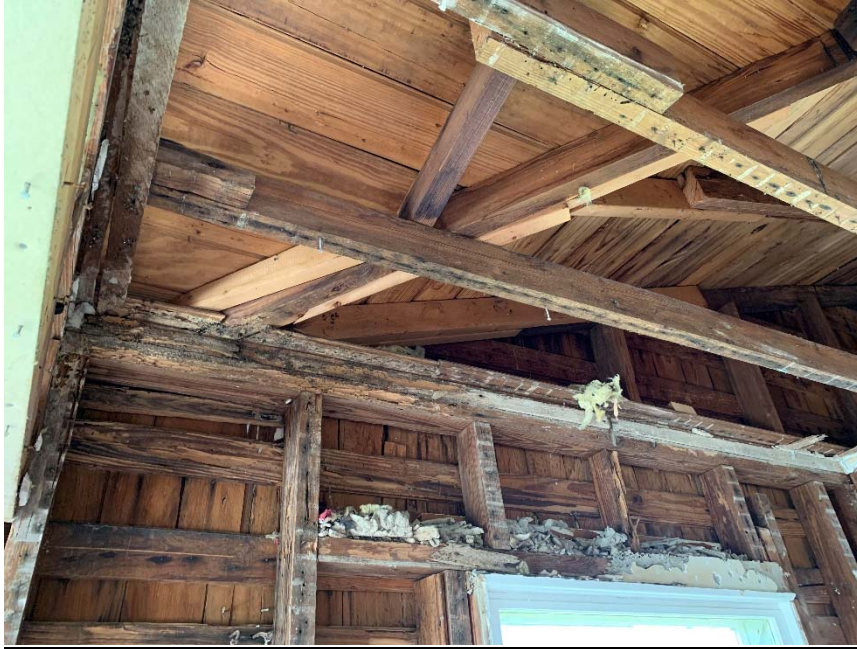
(Pic 9 East Hipped Roof – junction at Main Roof – Fascia damaged/misaligned w/Hipped Roof)
