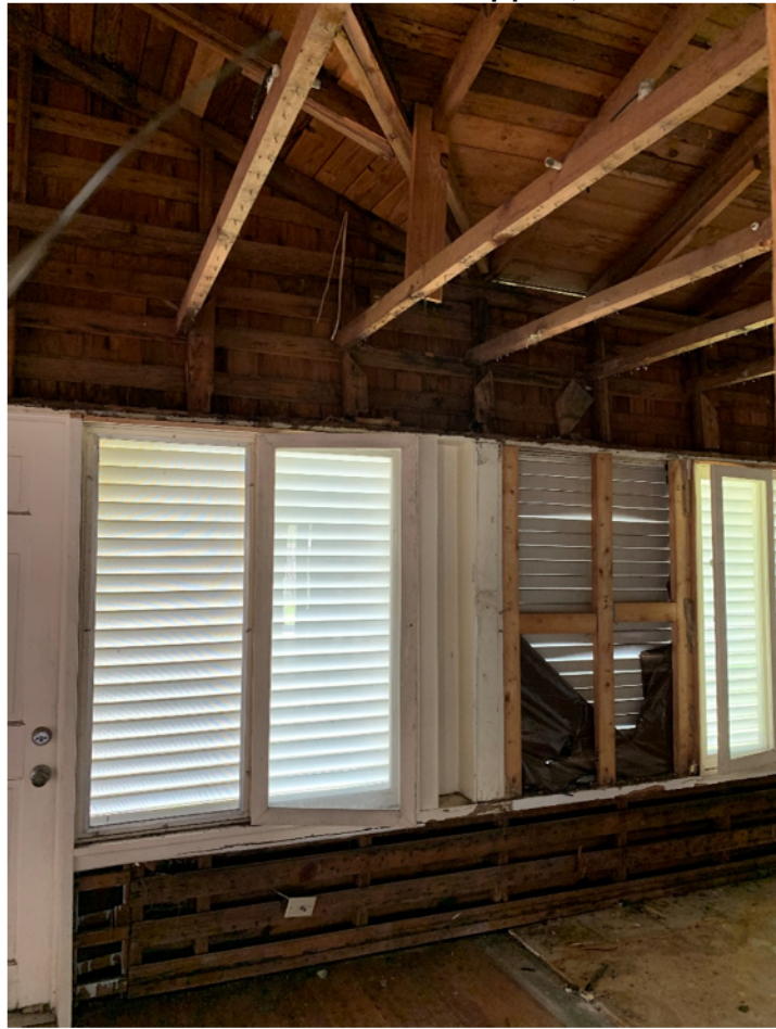
(Pic 4 – Junction Main Roof/West Gable at Exterior wall – note vertical support)
