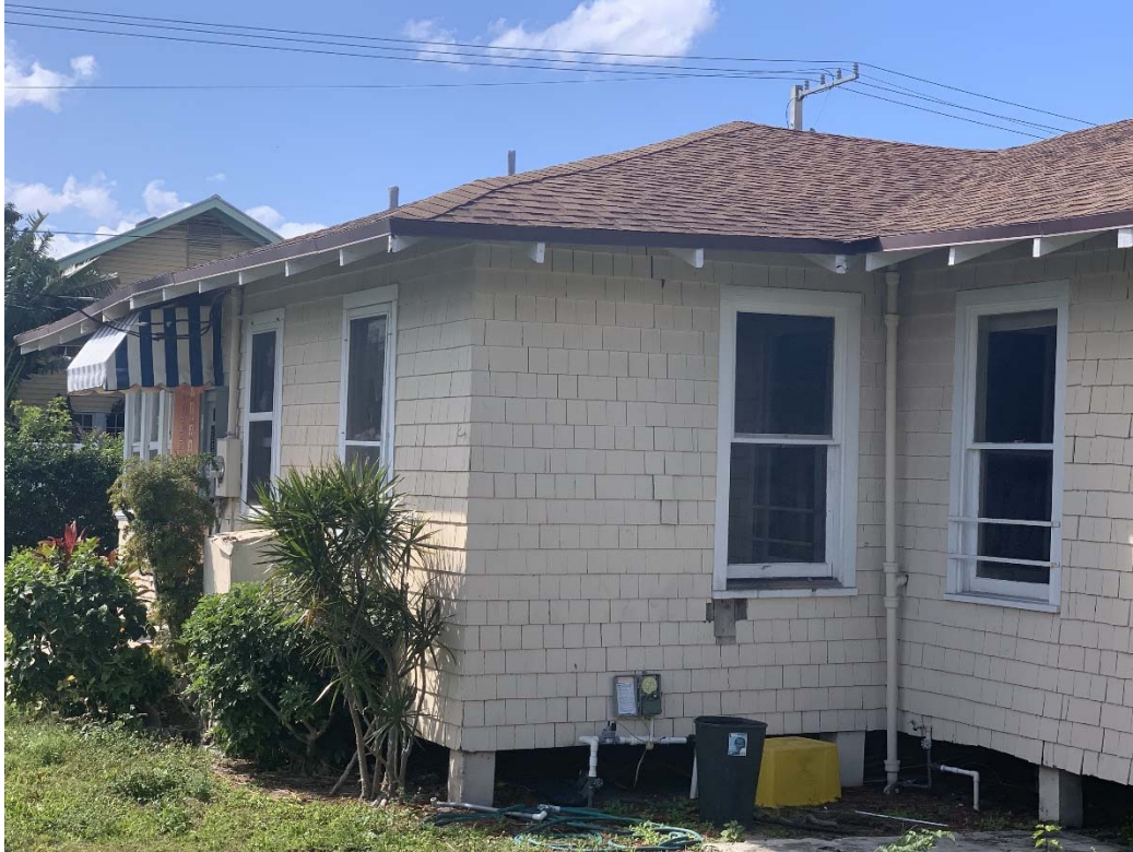
(Pic 11 East Hipped Roof Deflection)
