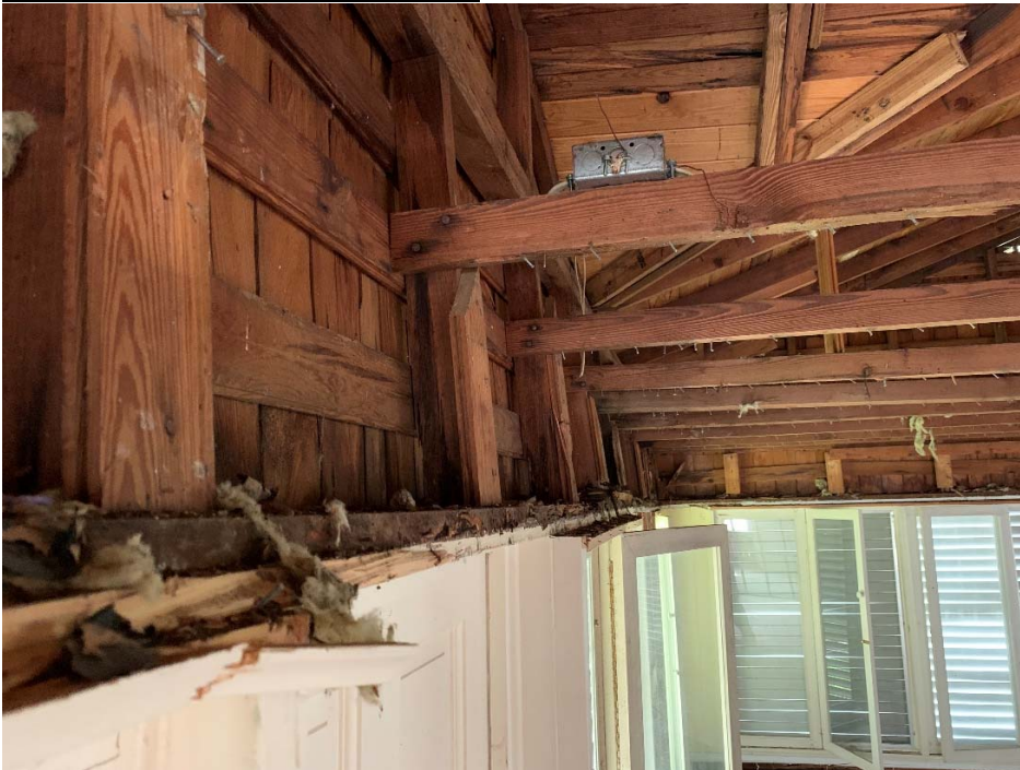
(Pic 5 – South Wall Pushed Out)
