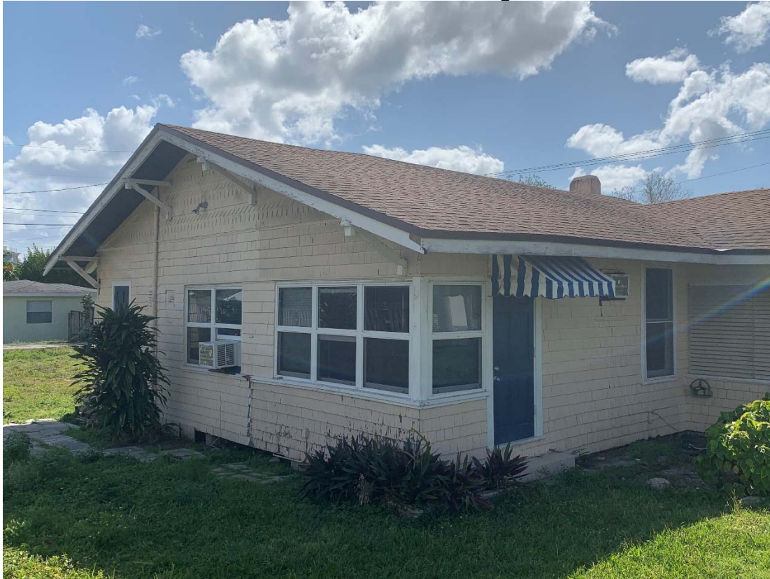
Pic 14 – North Gable Exterior Deflection – note deflection at Junction of Original North End Gable and Addition as well as deflection along the fascia
