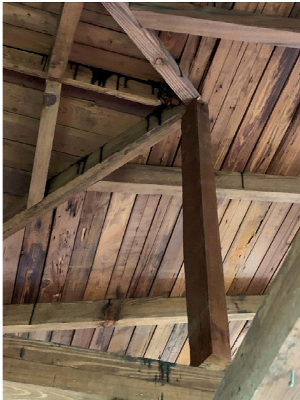
Pic 16 – Unsecured Vertical Support at Junction of two Roofs
