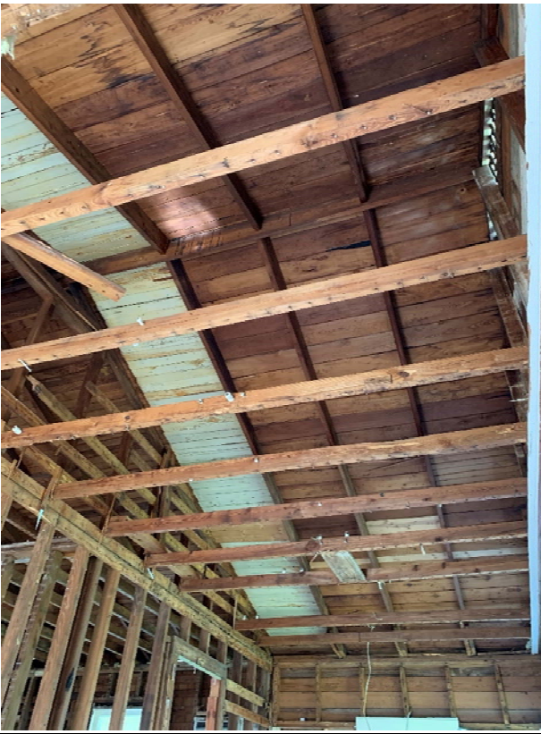
Pic 12 North Gable Addition – Ridge Beam
