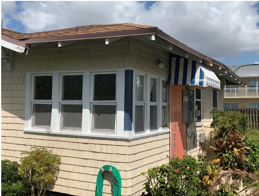
(Pic 9 East Hipped Roof – junction at Main Roof – Fascia damaged/misaligned w/Hipped Roof)
