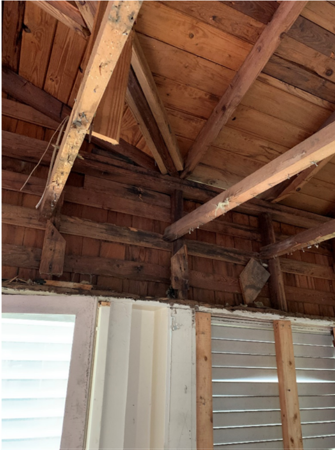
(Pic 5 – South Wall Pushed Out)
