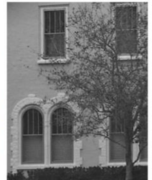
Flat and arched double-hung sash windows on a Mediterranean Revival house
