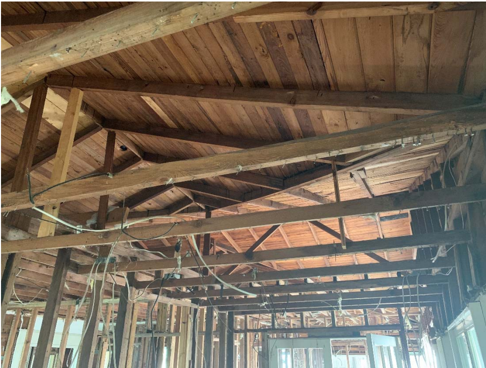
Pic 18– Randomly Placed Vertical Supports
