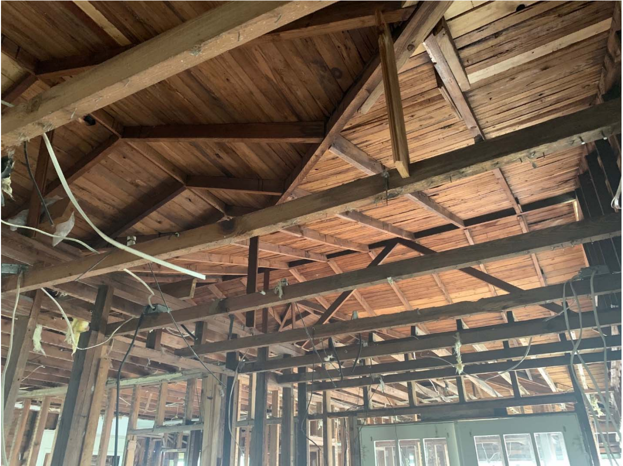
Hand framed roof framing without hurricane clips.
