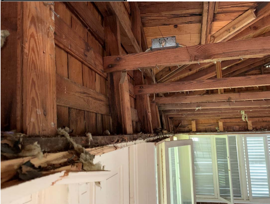
(Pic 5 – South Wall Pushed Out)
